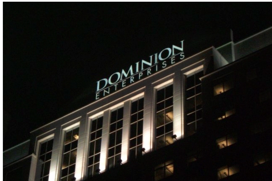
Daytime and nighttime views of the high-rise project in Norfolk, VA.
