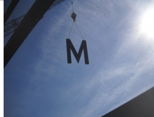
Top: Weather balloon used for sighting a hospital's new sign location; Middle Left: Scissors lift holding prototype letter in front of new high-rise building; Middle Right: Finished product installed; Bottom: Hoisting a new LED-filled letter after prototype approval.
