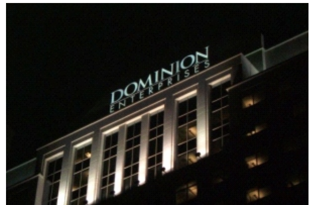
Clients at Norfolk's Dominion Enterprises' corporate headquarters chose Holiday Signs' plan to engineer infrequent and easy to accomplish maintenance into their sign project's design.
